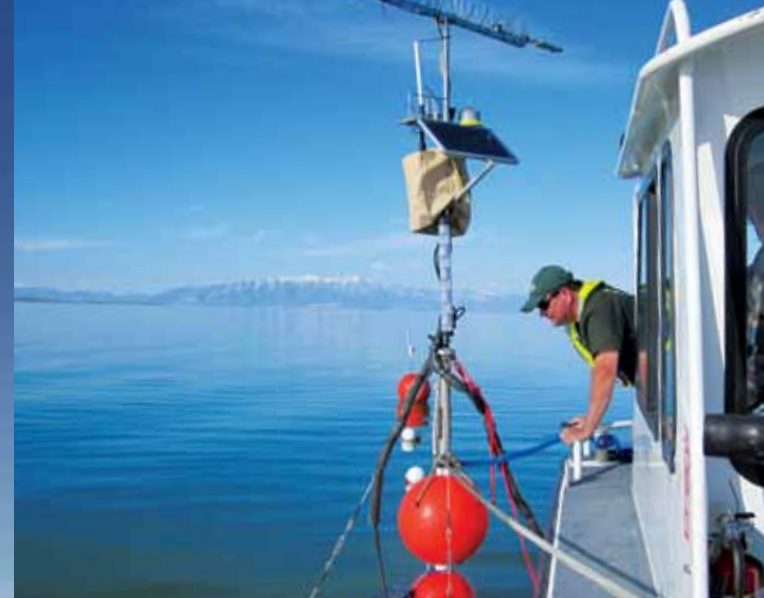
Completing installation of the LakeESP platform.
