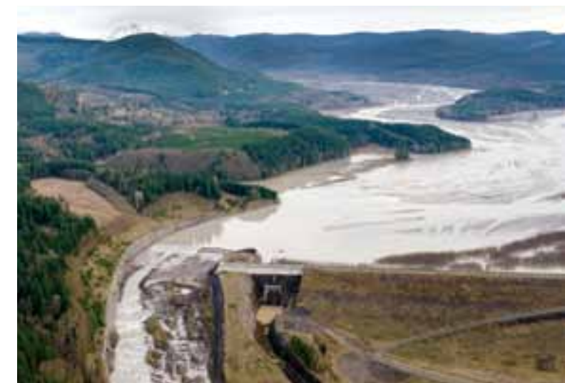
The Sediment Retention Structure on the North Fork Toutle River.
