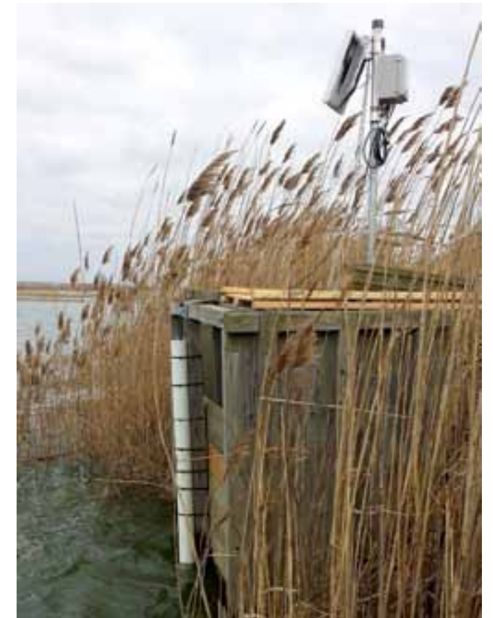
The monitoring system included a YSI EXO2 multi-parameter sonde and a NexSens 3100-MAST data logger with cellular telemetry.
