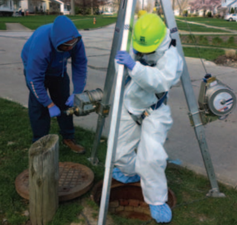
Left: Northeast Ohio Regional Sewer District, Installing flow meters in stormwater manhole in Parma. Right: Flowmeter on it's hanger. The probe is 10-15 feet down, installed in sewer district in Parma.
