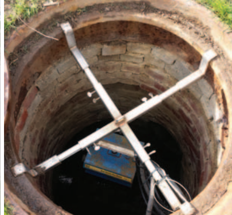
Left: Northeast Ohio Regional Sewer District, Installing flow meters in stormwater manhole in Parma. Right: Flowmeter on it's hanger. The probe is 10-15 feet down, installed in sewer district in Parma.
