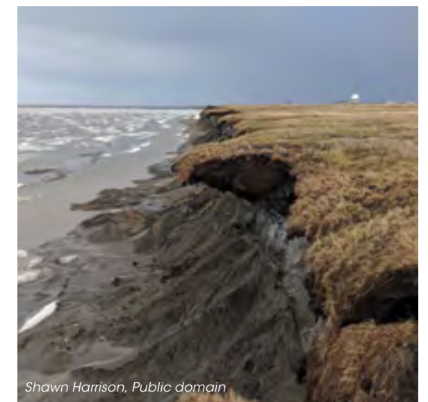
University of Wisconsin-Madison (2019) As Lake Michigan rises, bluffs collapse and geologists explore (News Article) Retrieved from www.news.wisc.edu/as-lake-michigan-rises-bluffs-collapse-and-geologists-explore/
