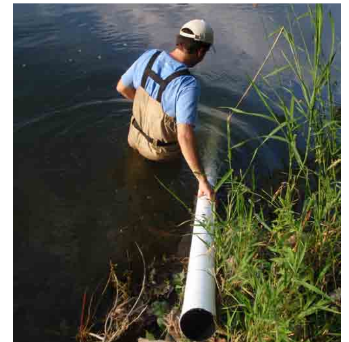
An SRBC field technician installs a deployment pipe, in which a YSI multi-parameter sonde will be securely housed.
