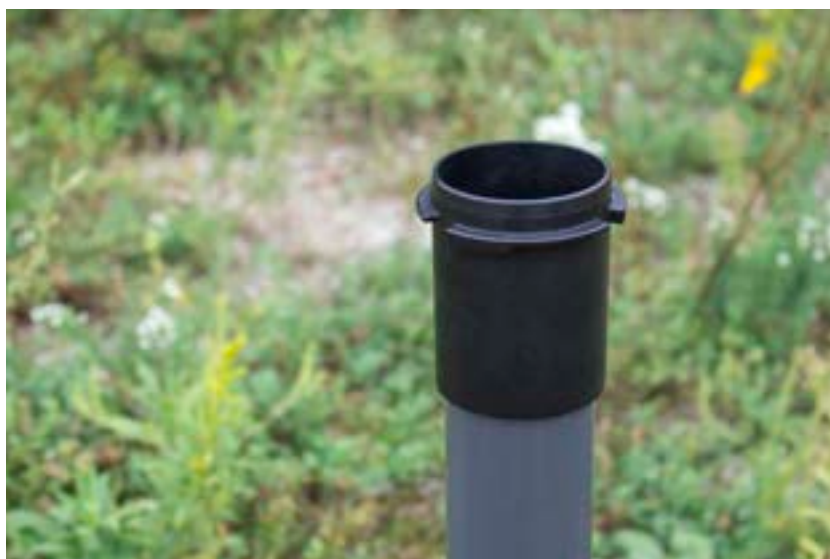
Figure 6-3 Install the Well Cap Base
