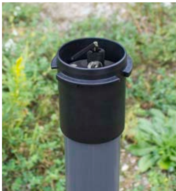
Figure 6-9 Install the Well Cap
